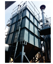
Pulse Jet Rectangular Bag Filters for Fine Dust Collection
